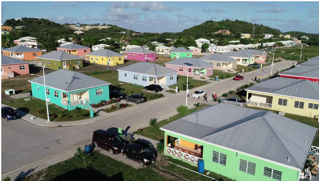
Pictures 9: Aerial Shot of Housing Development at Paynters
