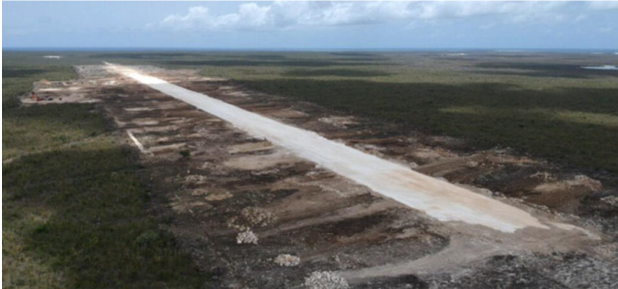
Picture 27: Preparatory Work at the New Runway
