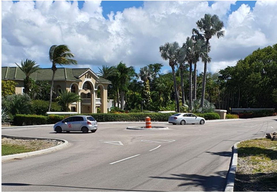
Picture 18: Road Improvement Work on the Sir George Walter Highway
