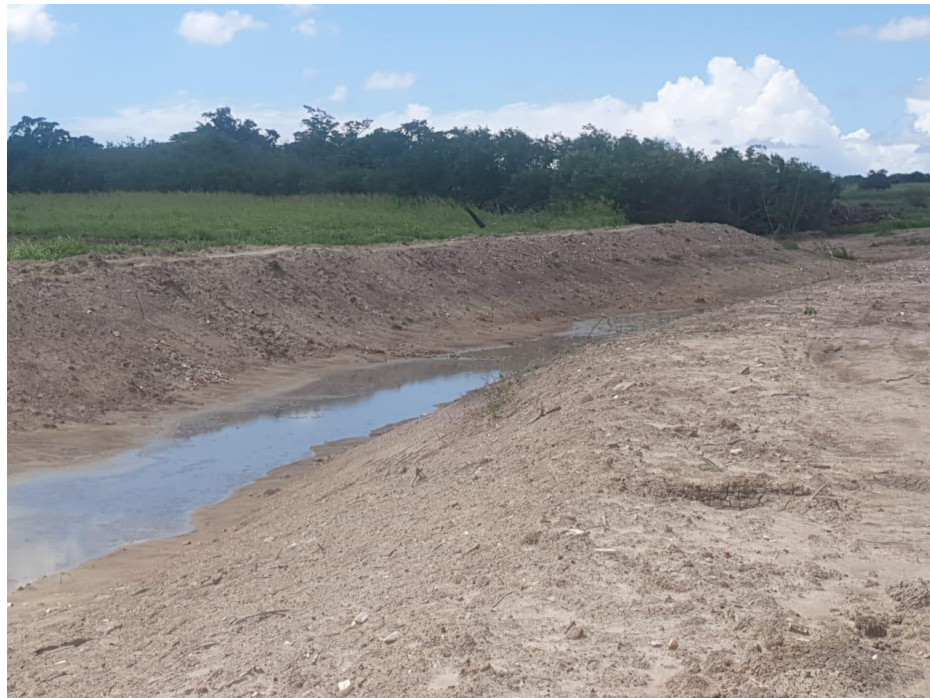
Picture 37: Dam Expansion Activities at Pares
