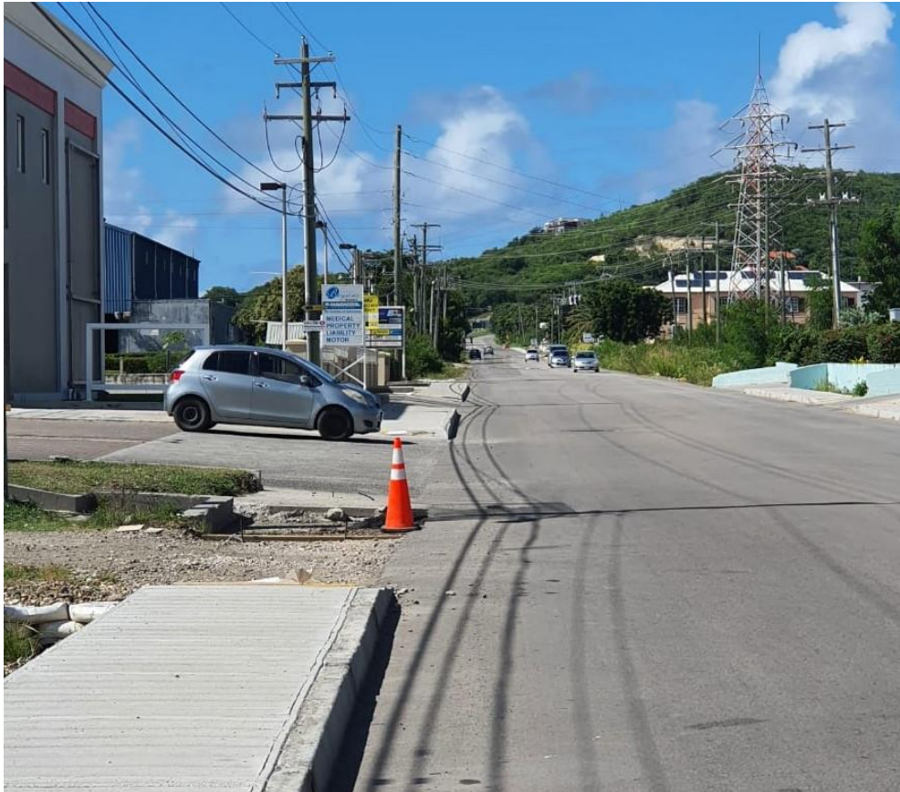
Picture 19: Completed Road Improvement Work on Friar's Hill Road
